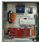
Motion 4000 cartop box with EMCO rope tension load weigher
